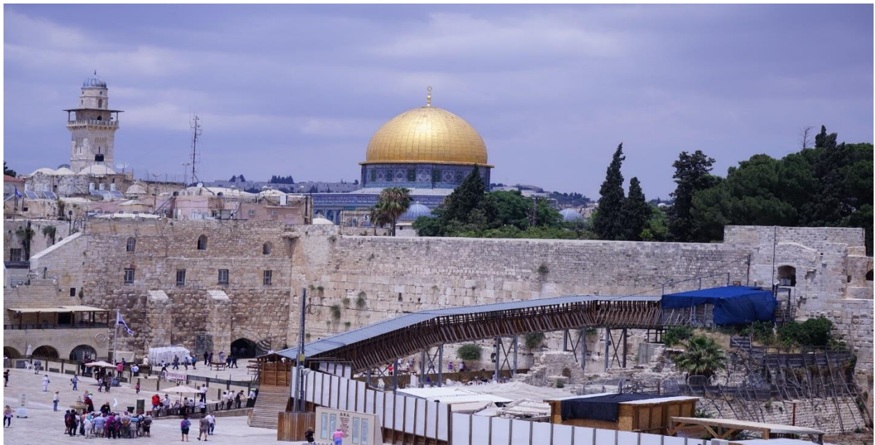
The Wailing Wall
